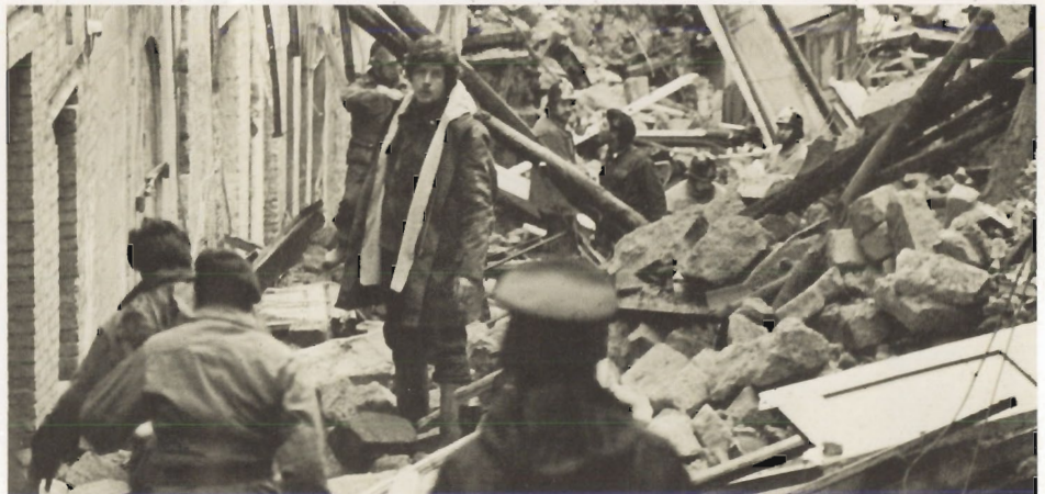
Workers continue to dig through rubble 10 days after the Italian earthquake.
